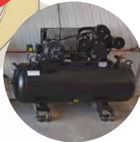
Compressed Air Used to remove water from around trims
